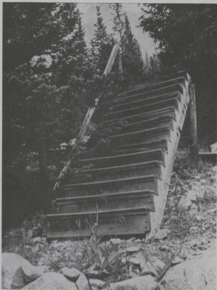
Old stairway at Hancock
