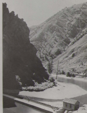
Gunnison River dam at East Portal. Intake of the 6-mile long Gunnison Tunnel (not shown) is to the right above the dam. The tunnel diverts water from the river to irrigate the Uncompahgre Valley.
