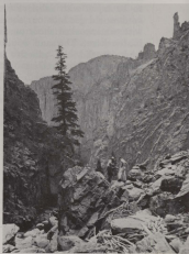
Davis and Fleming, in center, 3.2 miles below East Portal. Note driftwood in river channel.
