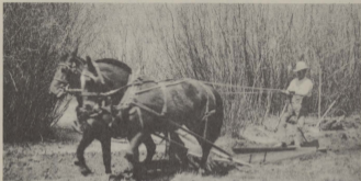
Martin Ditcher - Ranchers used this device to build irrigation ditches. Photo - Corb McNeill
