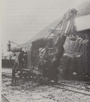
(Above) This narrow gauge one-yard air shifter seen at East Portal in August 1962 was one of the more exotic machines used by the tunnel contractors. First it arrived, it would have been a unique exhibit for any railroad museum. (Moffat Tunnel Commission) (Left) An unidentified Moffat Road 2-8-0 pushes an inspection train through the eastern part of the tunnel, prior to the installation of concrete lining. (Western History Collection, Denver Public Library)
