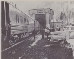
How many trains have penetrated the Moffat's darkness since 1928? The classic facade of the east portal looms over the waiting train and absorbs the people gathered to remember one of the significant events in Colorado history—the achievement of the dream of one of the state's most famous citizens, David H. Moffat. In the background, falling snow engulfs the silent mountains. (Charles Albi)
