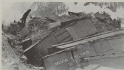
The Moffat scooters were involved in several runaways during the years of operation over Rollins Pass, and after the opening of the tunnel, the 215 took one more run. While ascending at East Portal on November 5, 1855, thirty-nine loaded coal cars got away from her, and she was running in excess of 40 mph before overturning near Rollinsville. Engineer Burns was injured as he jumped from the cab. A D&RGW wrecker had plenty of work to do the next day, but the 215 survived to become Rio Grande #6271 after the 1847 merger. (Otha C. Perry — Denver Public Library)
