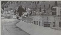
Western slope water flows from the east portal of the pioneer bore immediately south of the railroad tunnel. (Kenton Ferrett)
