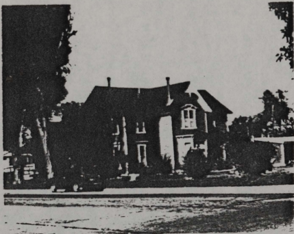
Figure 27: Gothic Revival residence in Gunnison. Centuries negative no. 102a-79-138.
