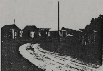
Figure 43: Hobo Junction. An overview of the cabins and shacks. View is to southwest. Centuries negative no. 102a-79-388.
