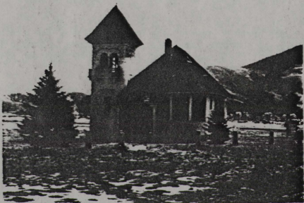
Figure 40: Paragon School. An unusually elaborate one-room schoolhouse. Centuries negative no. 102a-79-583.
