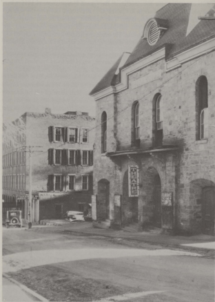
The Opera House in decay. Photo taken in the late 1920's or very early 1930's. The musician's balcony above the main entrance is almost completely deteriorated, the ornamental ironwork on the rooftop gone. The open windows on the upper story would indicate the building was probably in use at the time. The little white house, however, has vanished.
