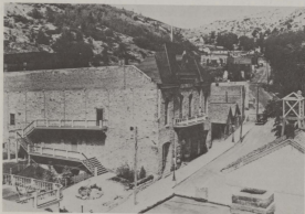
The Opera House in splendor in the late 1930's or early 40's — set off by the garden and Spanish arrastras which replaced the little white house between the Teller House and the Opera House. Observe the small pine tree near the street between the telephone pole and the brick edge descending from the peak of the downward slanting roof on the Opera House front. It now reaches nearly to the top of the building.
