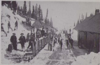
During the winter months it was necessary to use large crews of men to dig out the tracks from heavy snow falls and slides. The picture was taken at the Red Mountain depot looking north towards the Yankee Girl and Ironston during the 1890's.
