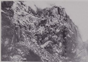
A two-engine passenger train enroute from Silverton to Durango paused near Rockwood long enough for W. H. Jackson to photograph it — probably around 1890. This was one of Jackson's more famous railroad pictures. The ledge for the track bed was cut from solid rock by men using hand held steel and black powder. (Library, State Historical Society of Colorado)
