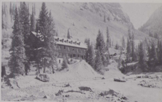
The abandoned boarding house alongside the Animas River just above Eureka as it appeared during October 1971. Massive three and four story boarding houses such as this were once commonplace throughout the San Juan Mountains, and were often the only home that an older, single miner might have. Some boarding houses allowed limited gambling, others did not, but all banned liquor. (Jack L. Benham Collection.)
