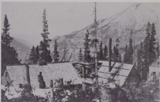
1888 Jackson photo of the Old Lout mine, showing upper shaft workings which were later abandoned when a tunnel was driven from a lower elevation in Poughkeepsie Gulch. Between 1876 and 1888 the mine produced around $400,000 worth of rich silver ore. (Denver Public Library, Western History Department)
