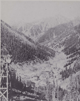
The Gold King Mill and Gladstone as it looked around 1906 from mid-point on the Gold King Tramway. The tramway continued on up the mountain to the main adit (12,000 feet in elevation) just below Bonita Peak and was capable of running 300 to 400 buckets, each carrying 700-800 pounds of ore per day. The tracks of the Silverton, Gladstone and Northerly can be seen winding down Cement Creek. The two large multiple story buildings in Gladstone were boarding houses. The Gold King Mine also had a "Typical San Juan" 4-story boarding house at the main adit level. The Mogul Mill is to the right of town and partially hidden by the trees.
