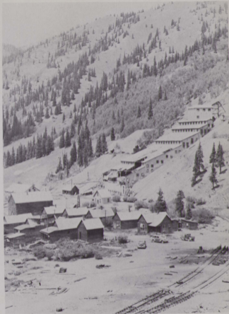
The Mogul Mill was built in Gladstone around 1904. A one and three quarter mile aerial tramway connected the mill to the mine adit located south of Hurricane Peak at an elevation of 11,400 feet. At the time of this photograph (late 1930's) the mill had been abandoned and the town of Gladstone was in various stages of disrepair. The tracks of the Silverton Northern (formerly SG&N) had not been used since 1924. The repeated flooding of Cement Creek had covered the tracks with silt and debris.
