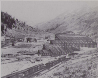
The imposing Gold Prince mill, one of the largest in the state, dwarfs Animas Forks and the valley in this 1905 photo. Two miles of rugged mountain terrain separated the mill from the mine. The aerial tram went up the left hillside.
