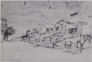
Burros loaded with track iron for mines near Silverton. The burro behind the gentleman on the left is carrying the bin portion of an ore car. Picture taken on 13th Street around 1900. (Denver Public Library, Western History Department)
