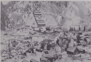
Eureka in the 1920's. The "new" Sunnyside mill completely dominated the town. The aerial tram to the mine paralleled the canyon to the rear left. Steel for the mill was obtained from the abandoned Gold Prince mill at Animas Forks.
