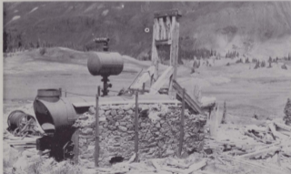
A Mineral Point mine as it appeared in August 1971. It was common practice for the miners to place a reinforced rock wall around steam boilers to conserve heat and serve as a barrier in case of boiler explosion. The wooden headframe above the shaft can be seen immediately behind the boiler. A steam operated winch lies rusting in the rarefied atmosphere on the picture's left. The present day jeep trail from Ouray and the Million Dollar Highway up the canyon of the Uncompaghre to Engineer Pass and Animas Forks, lies in the canyon to the rear of the picture. (Jack L. Benham Collection)
