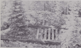
Otto Mears' turntable on Corkscrew Gulch as it appeared in September 1975. The main line from Silverton approached the table from the left or south and departed on the barely discernible track bed to the left rear of the photograph, and on to the Silver Bell mine, Ironton and Albany. Aspens and 50 year old spruce trees have all but obliterated traces of the railroad bed by growing up between the ties.
