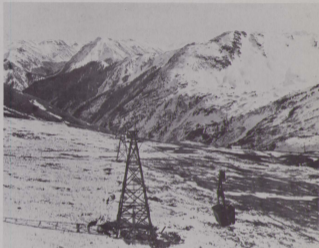
A three mile aerial tramway line connected the Sunnyside mine to the Eureka mill which was about 2000 feet below the ore loading terminal at the mine (elevation 12,300 feet). The tower in the foreground was 80 feet high and the buckets held about 1300 pounds of ore. Each bucket made the six-plus-mile round trip in about 75 minutes.
