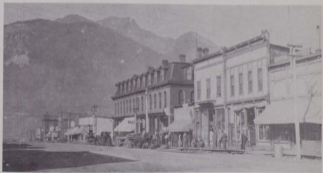
Silverton's Main (Greene) Street about 1909. The Hub Saloon was operating in the Grand Hotel building as a stage coach was unloading passengers. With the exception of the horses and canvas awnings, the buildings haven't changed much the past 68 years.
