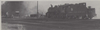
Engine #487 getting up steam in the Chama, N.M. yards early in the morning. An electric fan mounted on the smoke stack creates additional draft in the boiler.
