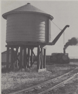
The water tank at Antonito, Colorado.
