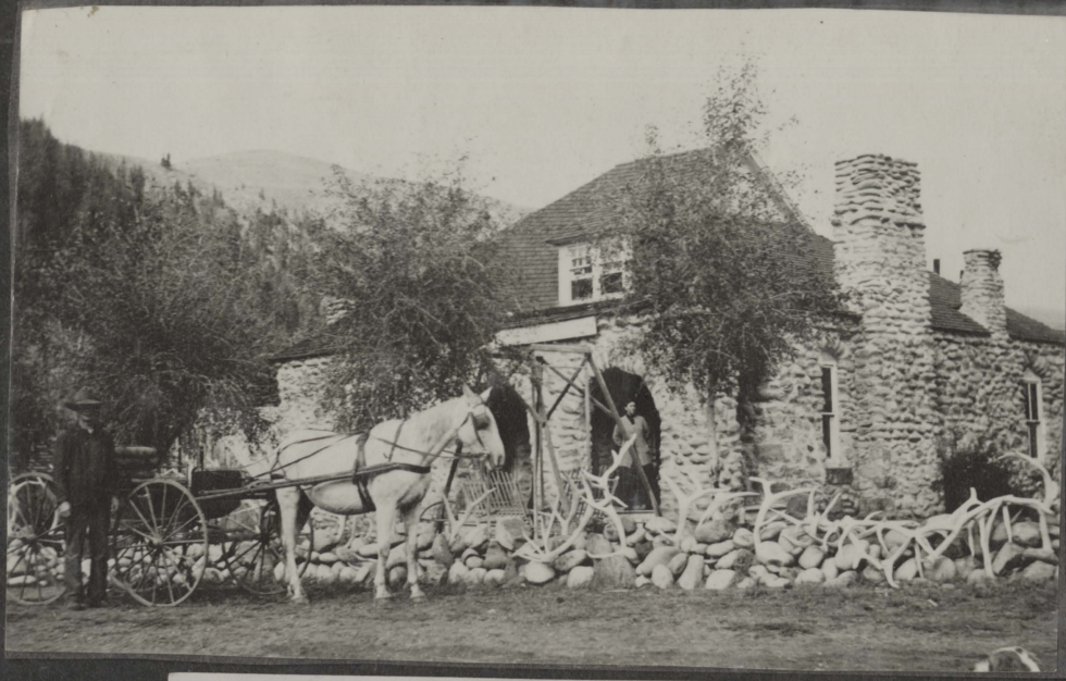
Lodge at Almont Destroyed by Fire
