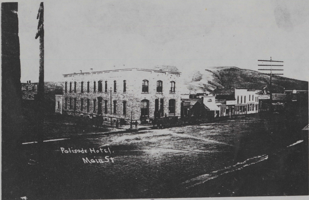
Called Tabor - then Palisades Hotel - Corner Main and Virginia, Destroyed by fire. Basement hole remained into 1930's, Built 1882
