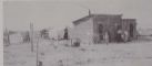
The Freeman place in Appleton is shown here in 1903. The family moved into the cabin in 1895, and, like many others, were waiting for completion of the Highline Canal.
