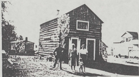
512 N. TAYLOR 1936 BEFORE REMODELING BY JOHN PECK McCreery Ranch House
